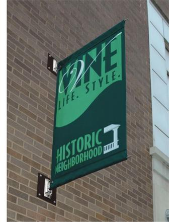
Because the wall is not designed for this type of concentrated force, there is a tendency for the outer edges of the main casting to quickly wear into the surface. This happens through constant motion of prevailing winds and slight movement of the main casting. While this vibration has little effect on the typical street pole installation, it will eventually wear and loosen the wall-mounted installation. The looser the installation becomes, the quicker it will fail.
